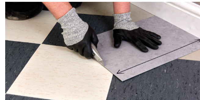
Figure 4.8 Cutting the perimeter tiles (diagonal cut)
