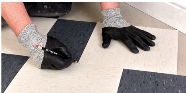
Figure 4.7 Marking the perimeter tiles (diagonal cut)
