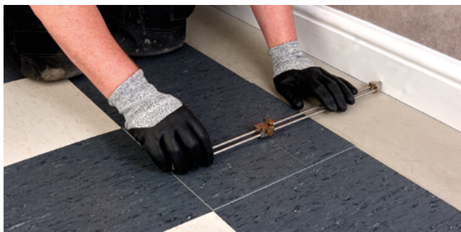
Figure 4.6 Measuring a tile using a scriber
