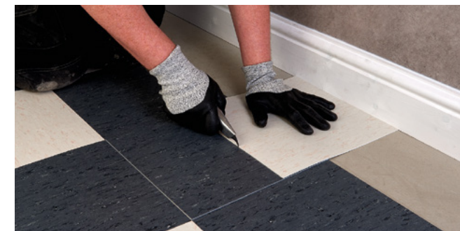
Figure 4.5 Measuring using an overlapping tile
