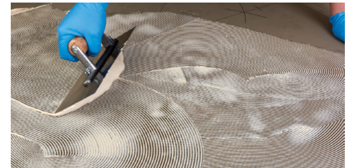
Figure 4.10 Selection of the correct adhesive is essential
