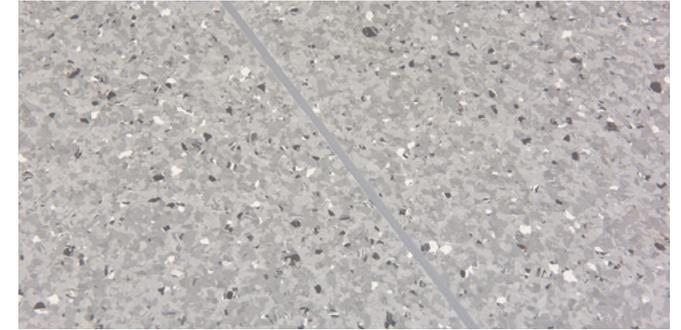
Figure 9.6 Final weld
