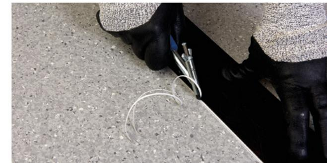
Figure 9.1 Grooving the seam
