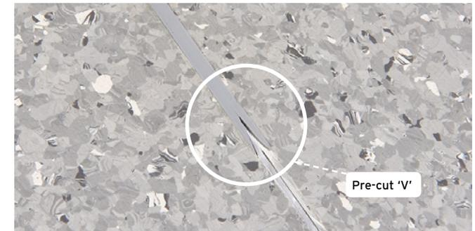
Figure 9.3 Weld joins
