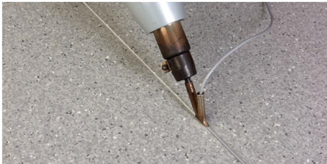
Figure 9.2 Applying the weld
